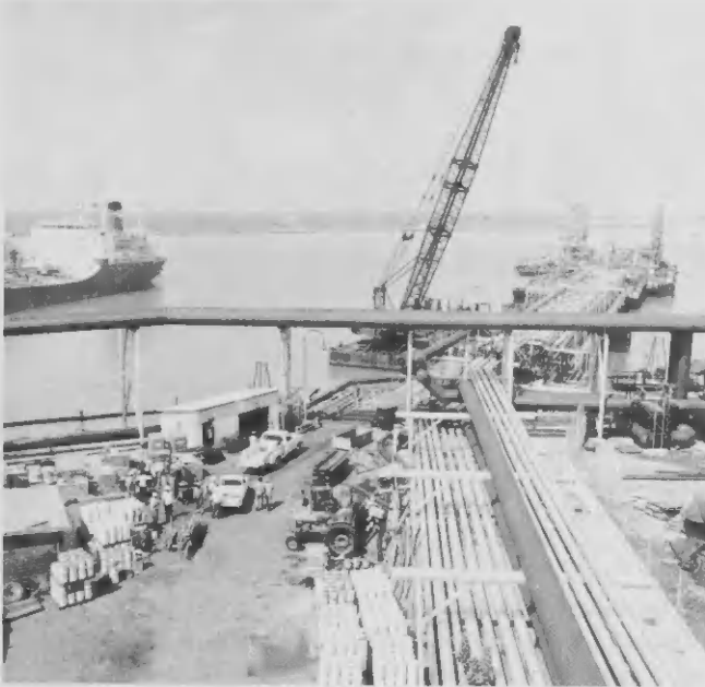
Huge crane and barge assist in recent No. 3 Finger Pier turnaround. Grua y "barge" grandi ta yuda den revision di Finger Pier No. 3.
